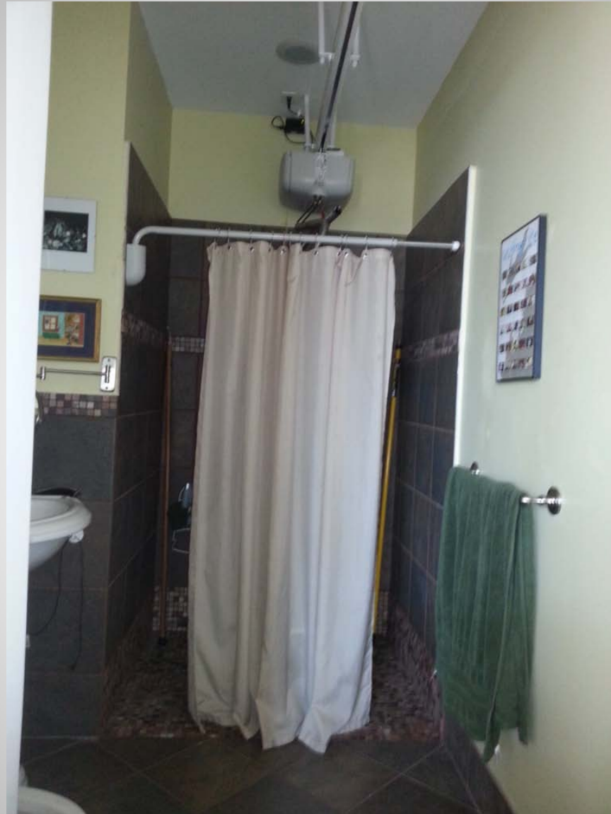
Mechanical Lift, Roll-In Shower
