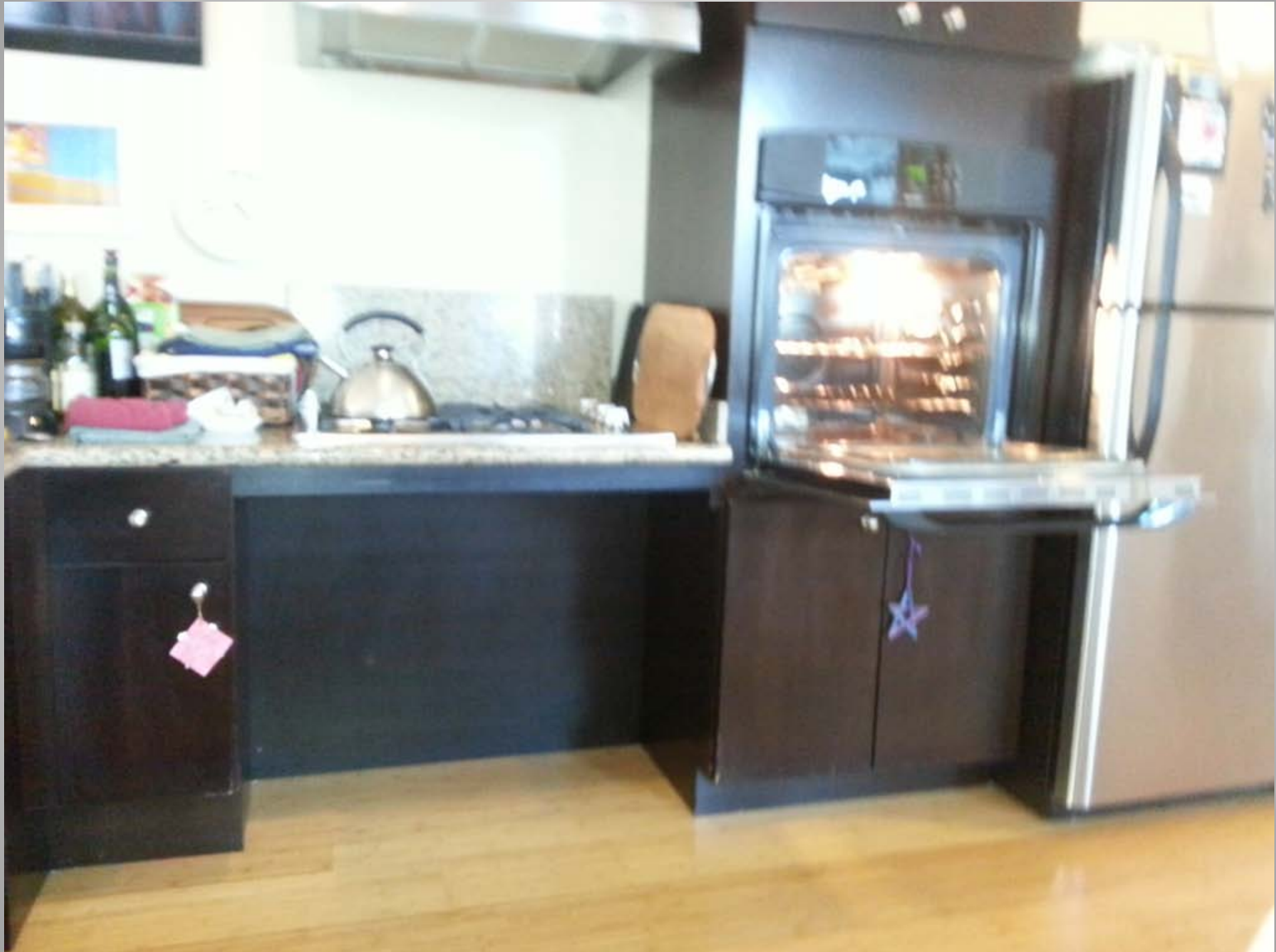
Wheelchair Access to Stove
