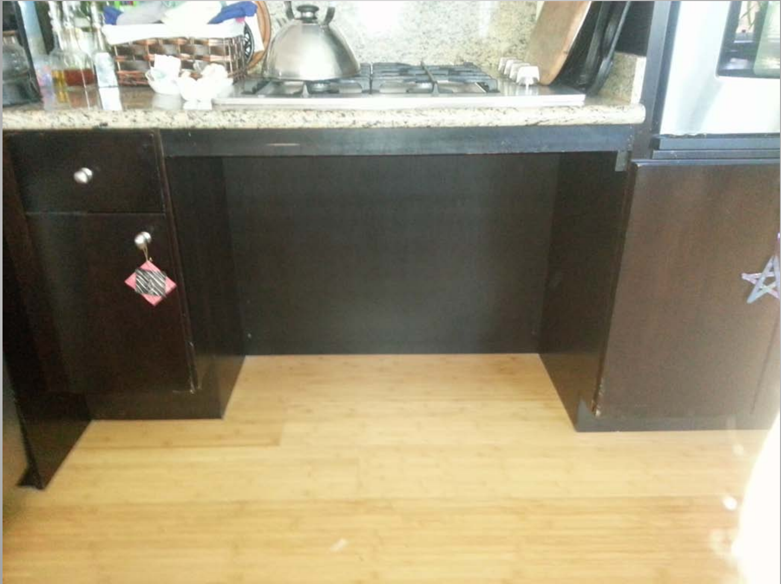
Wheelchair Access to Stove
